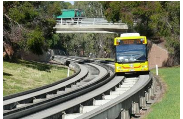
Figure 4: Samples of BRT running way types. TOP - mixed traffic running way; MIDDLE – at-grade median running way; BOTTOM – grade separated busway, Adelaide, Australia.
